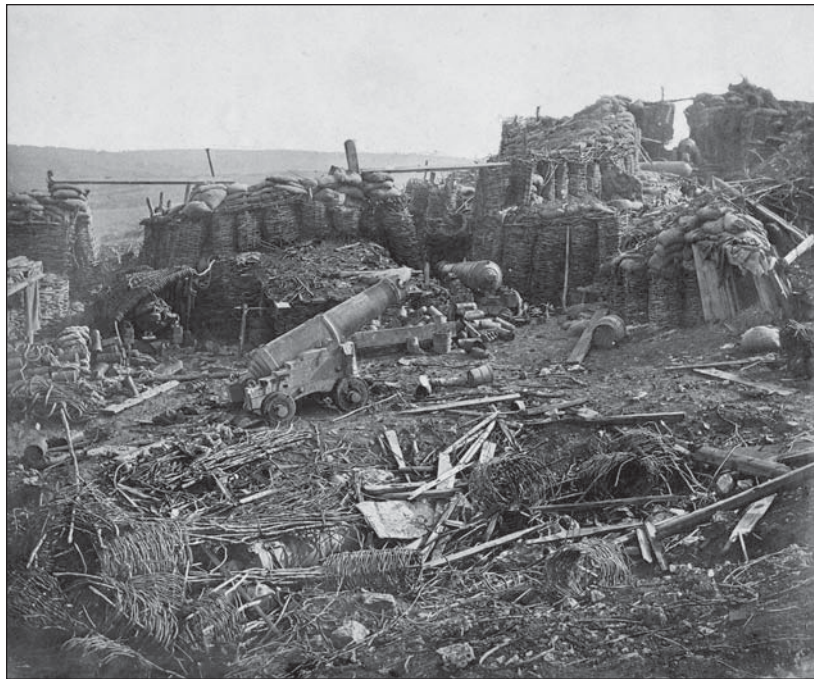
The aftermath of the British assault on the Redan, a large Russian battery, which contained several guns and was protected with sand bags and big round baskets stuffed with earth called “gabions.” After a three-day bombardment which saw almost 100,00 rounds of shot and shells launched on the Russian positions, the British briefly held it before being forced to withdraw after a Russian counter-attack. Photo James Robertson, 1855
